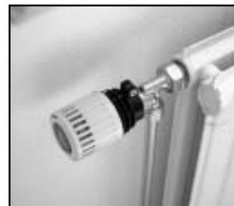
Open the thermostat valves completely.
